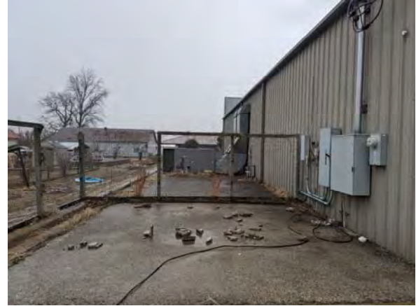
View Behind Structure
