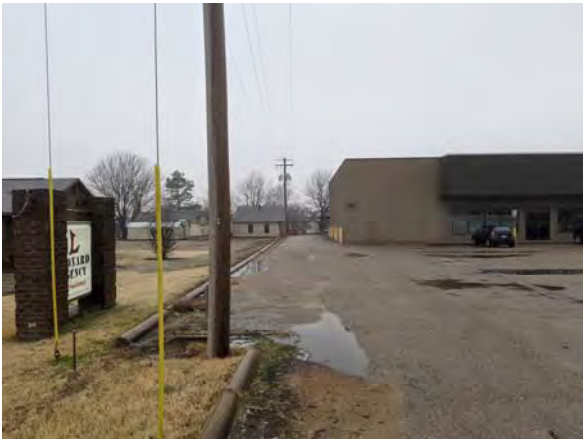
Southeast Corner Facing West
