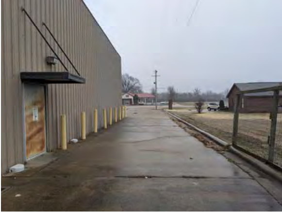
Southwest Corner Facing East
