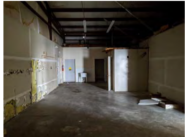
Interior Storage / Restrooms
