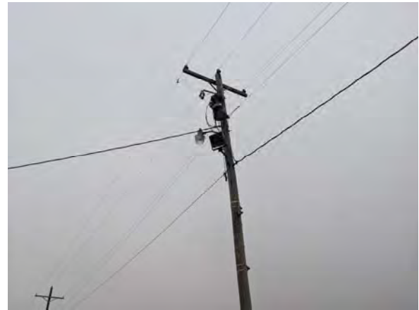
Pole-Mounted Transformer
